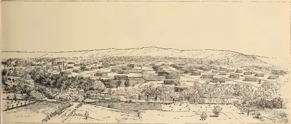
TANKS AT A STORAGE DEPOT.
